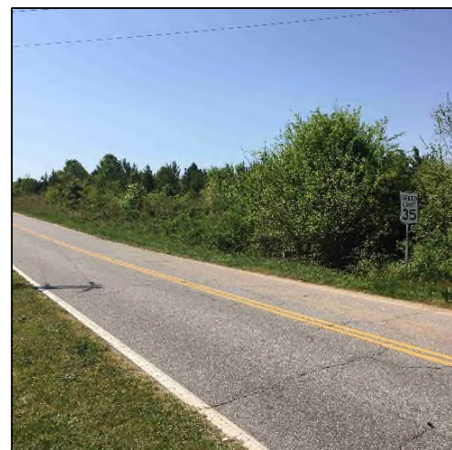
Site frontage from Salem Church Road
