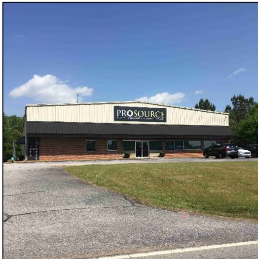
ProSource Plumbing supply
